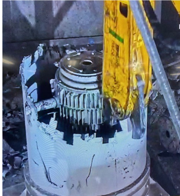
RB Air Cooler Demolition with Brokk 900
