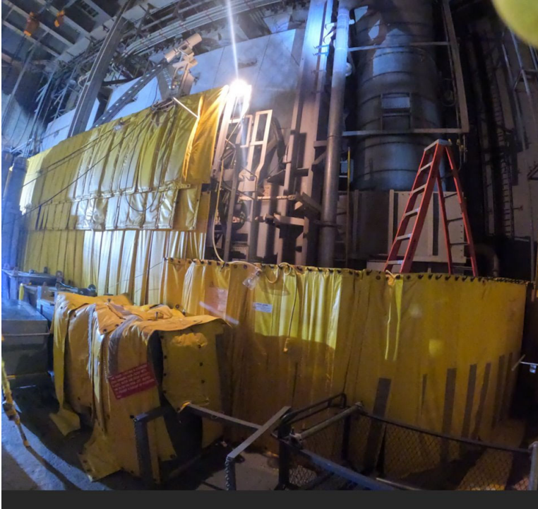
RB Air Coolers prior to Demolition with Brokk 900
