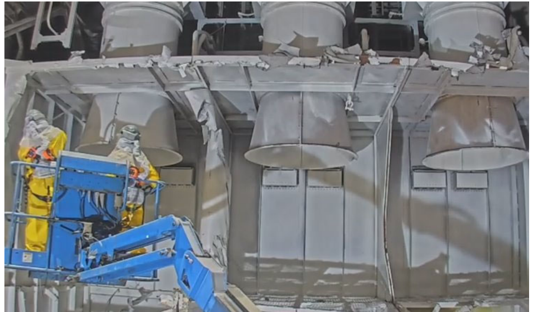
RB Air Coolers prior to Demolition with Brokk 900
