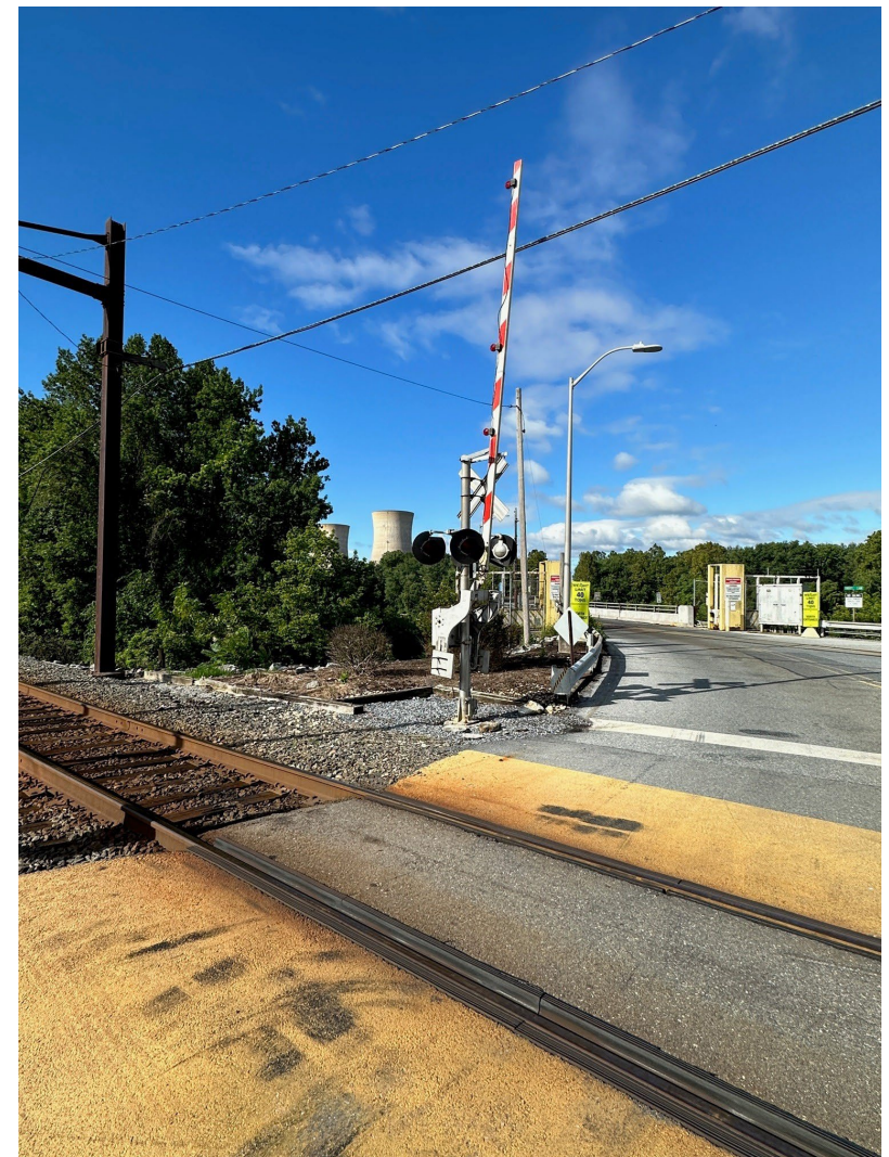
Railway at TMI at site entrance with overhead clearance considerations
