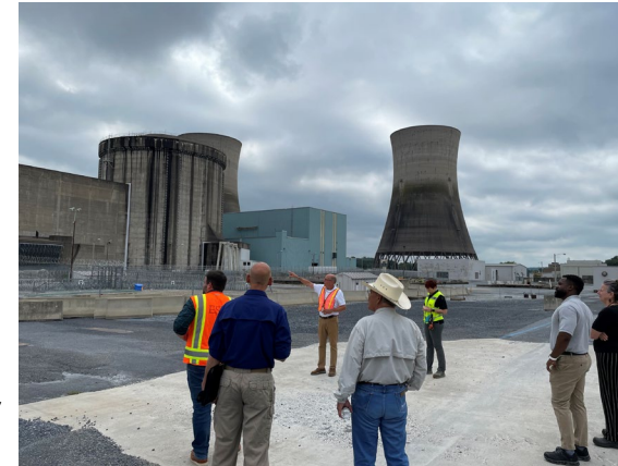
TMI-2 Reactor Building and Cooling Towers
