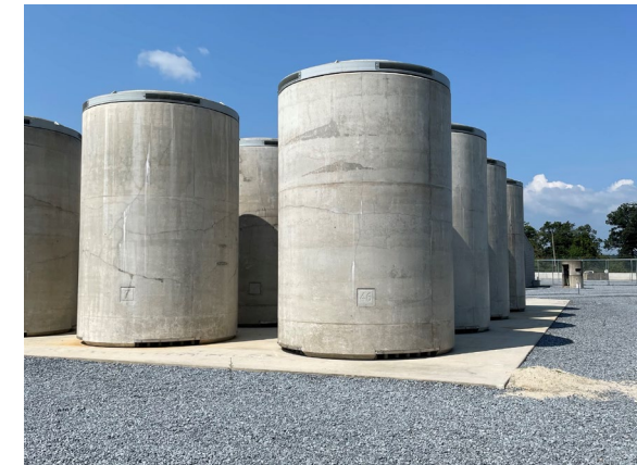
ISFSI Pad with Expansion Room for TMI-2 Casks
